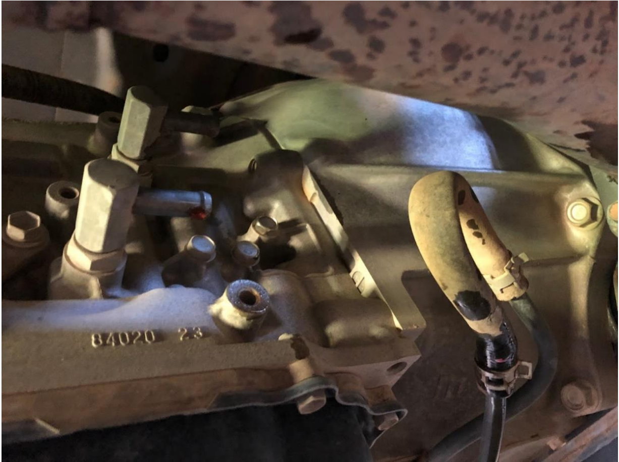
This image shows the use of the original hose to loop back to the original cooler
