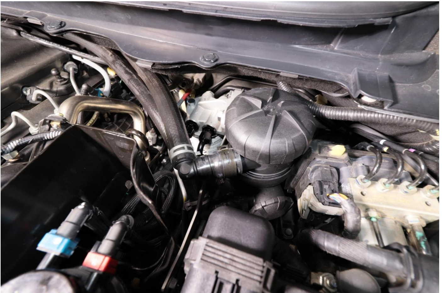
Completed installation of the ProVent® and PL150DP
