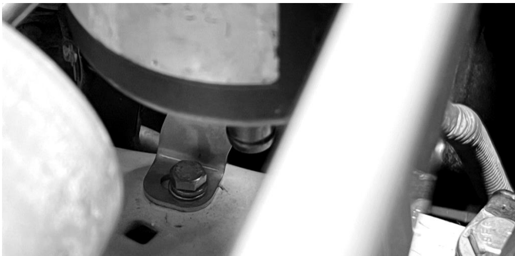
Brace lower mounting location, M6 hardware used to secure
